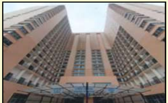
The 824-room capacity Hostel Block at ABVIMS and Dr. RML Hospital, was inaugurated by Hon'ble Union Minister of Health & Family Welfare and Chemical & Fertilizers on January 8, 2024
